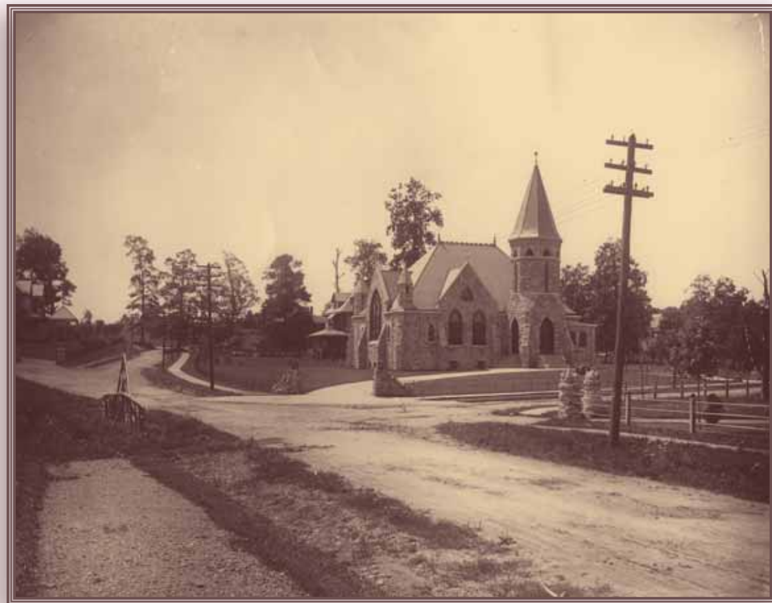
An early photo of the Wayne Methodist Episcopal Church, with unpaved roads. Note the bridge in the center left, showing the location of a stream now underground—and the source of perennial water problems for both the church and the middle school basements.
