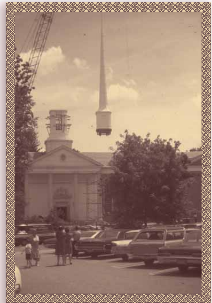
The steeple being hoisted into place, 1967.
